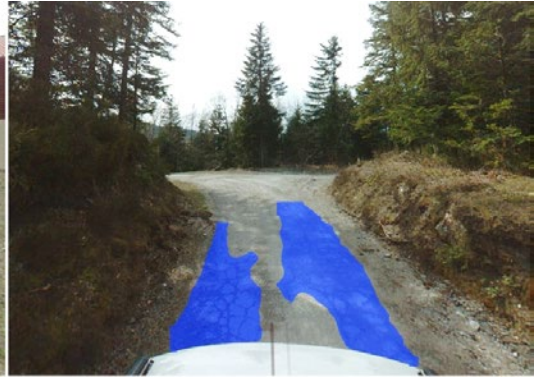
Road photo at station 2+406 showing pavement condition rated as 2
